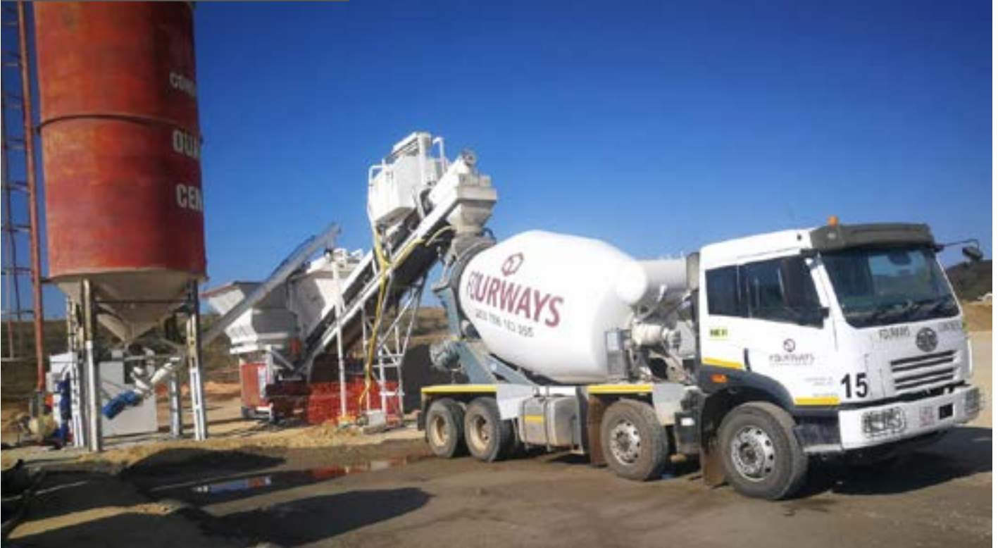
MIMOSA MINE PLANT
