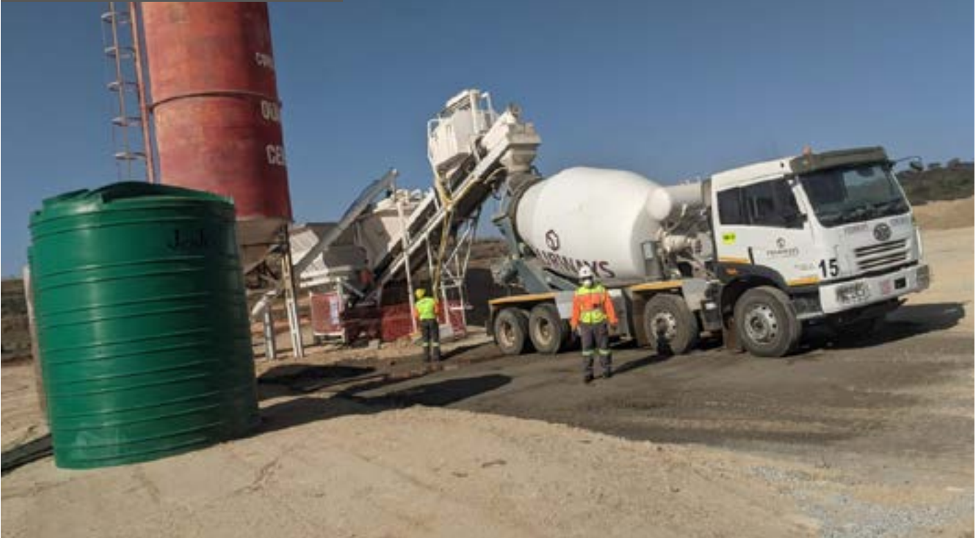
MIMOSA MINE PLANT
